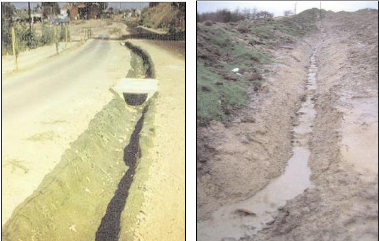
Figure 3 | Examples of Diversion Drains
